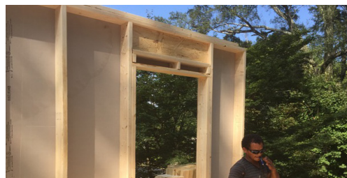
This recessed header allows for better insulation installation.
