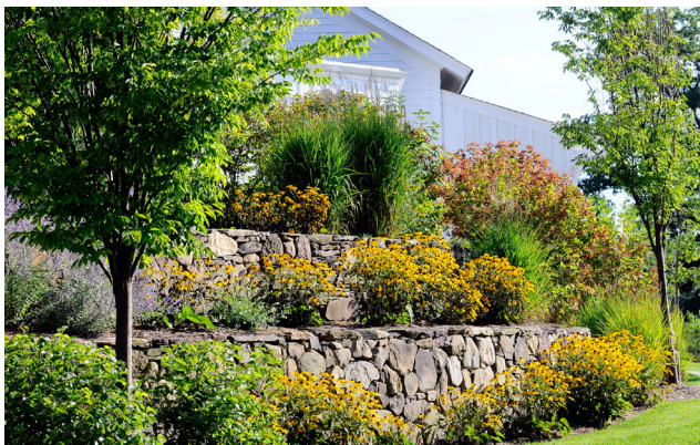
Neighborhood Center Retaining Wall
