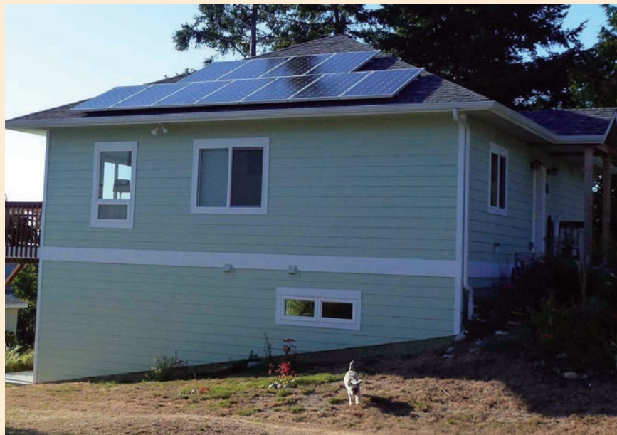
Solar panels can cover the entire electricity load of the home because of small details like using the slope of the site to allow daylight into the basement.
