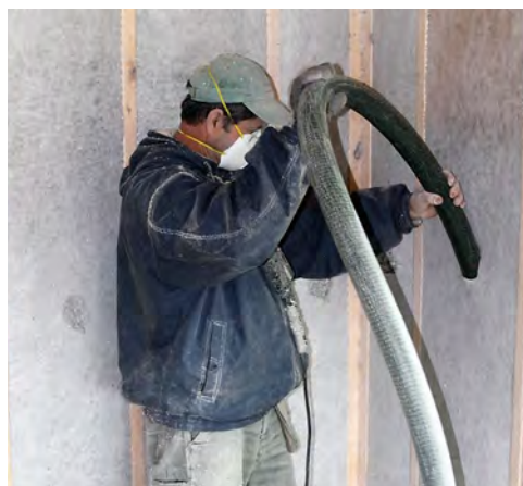
Photograph courtesy of Cellu-Spray Insulation
