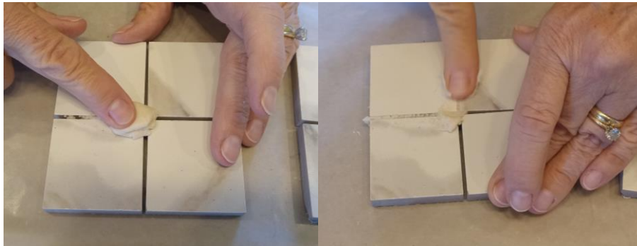
Figure 7. Force grout into spaces between tiles
