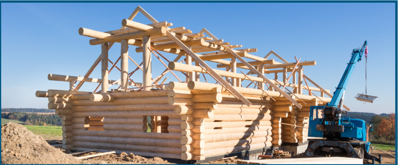
LOG HOME UNDER CONSTRUCTION
