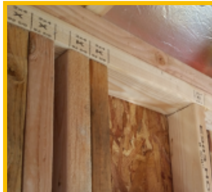
PRECUT WALL FRAMING
