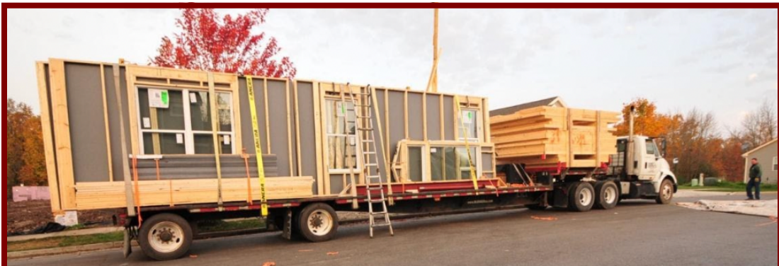
WALL PANELS BEING DELIVERED
