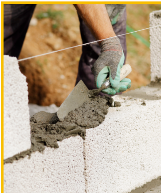
CONCRETE MASONRY WALL SYSTEM
