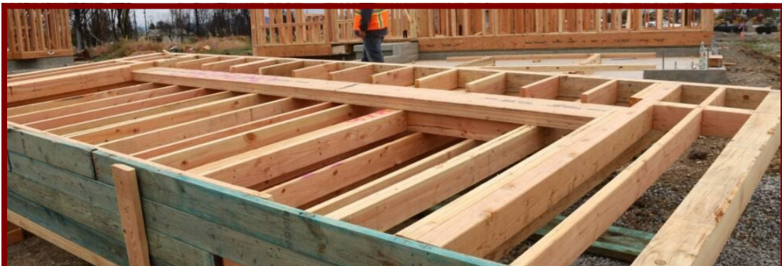
WALL PANELS ONSITE
