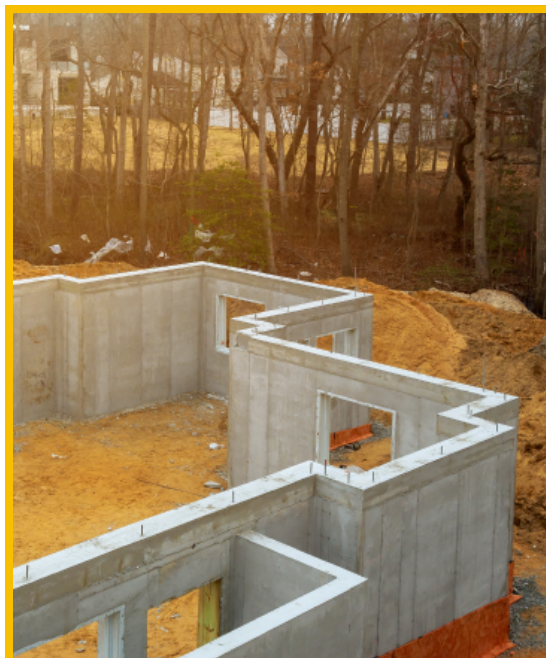
POURED CONCRETE WALLS
