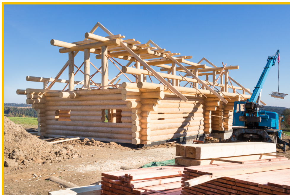
LOG HOME FRAMING
